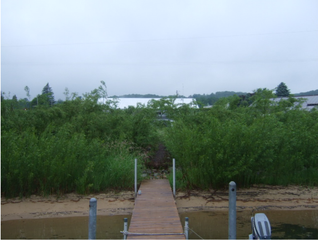
Photograph 1: Example of natural vegetation and stone shoreline protection. Vegetation holds shoreline in place in conjunction with coconut coir log and natural stone rip rap. After two to three years of growth rip rap and coconut coir log are not visible. View sheds are not maintained.
