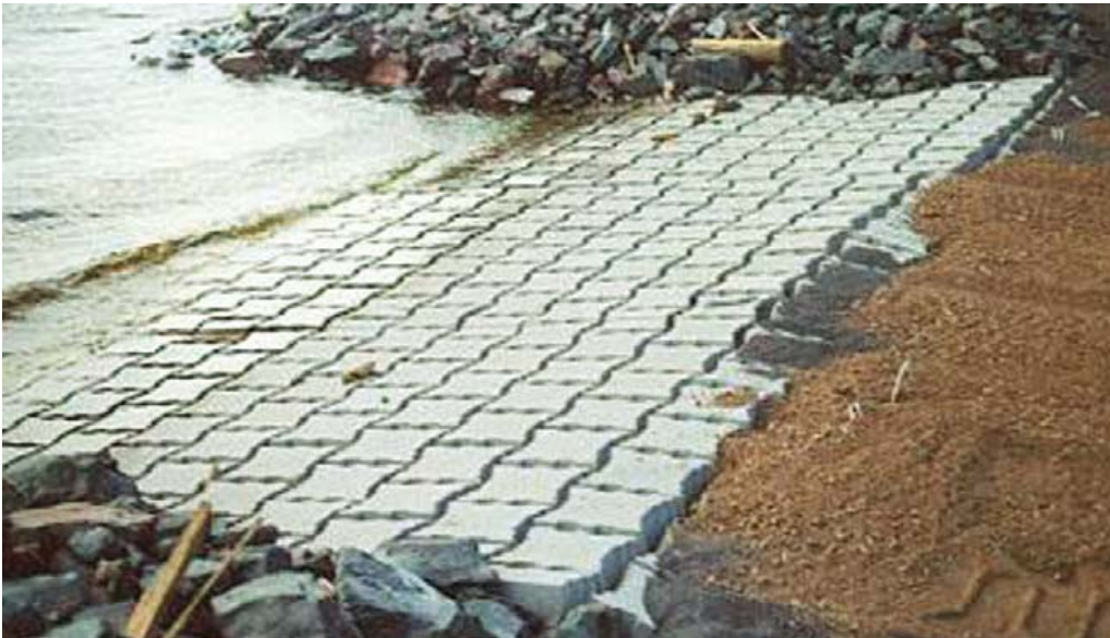
Photograph 2: Example of hard armoring of beach access location. This approach is suitable for areas that receive significant use from foot traffic and/ or launching small water craft. Size of access point can be tailored to specific use and need and incorporated into a more natural shoreline design. Alternatively, the block pavers in the photograph above can be replaced with large flat landscaping rock.
